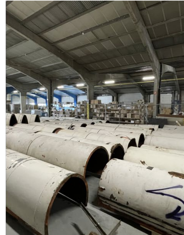
Pompidou: 3 ships of outside walls, to be cleaned & re-used
