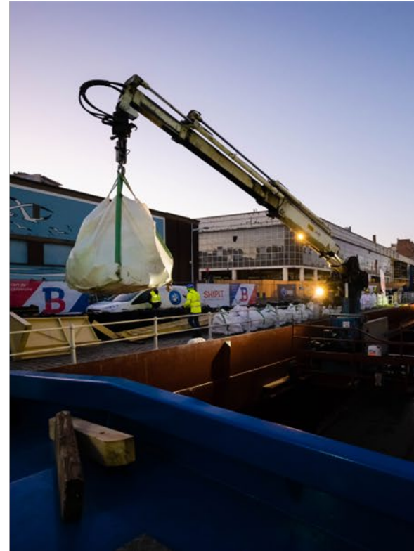
Pompidou: 3 ships of outside walls, to be cleaned & re-used
